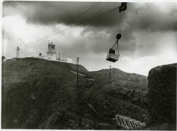
Transferring materials onto the island in 1965
